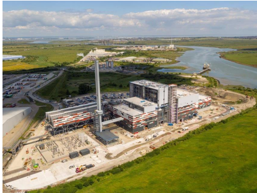
Figure 5.1 – K3 facility being constructed (July 2019)
